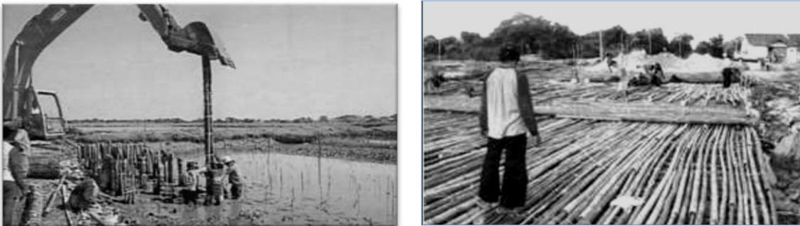
**Fig.2.** Pile mattress Bamboo for Toll Road Embankment Tambak Oso Surabaya [5].
