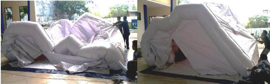
**Fig. 4.** Process Setting-Up Air inflated Structure
