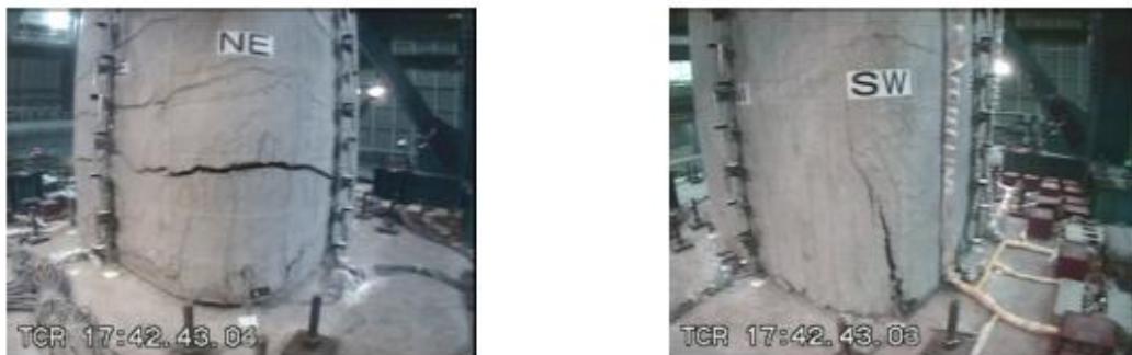
Fig. 6 Damage progress of C1-6 at the NE and SW corner during the 6th shake-table excitation
